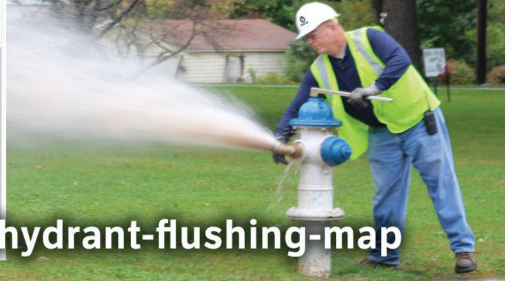
MPW's flushing procedure is a comprehensive maintenance activity that helps keep the water mains clean and provides valuable feedback on the condition of each fire hydrant connected to the MPW water distribution system. When MPW flushes hydrants in the spring and fall, customers can use our new interactive map to watch our progress and know when we'll be flushing in your area.
