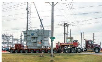
Contractors deliver the North Substation's new 161kV/69kV Auto Transformer
