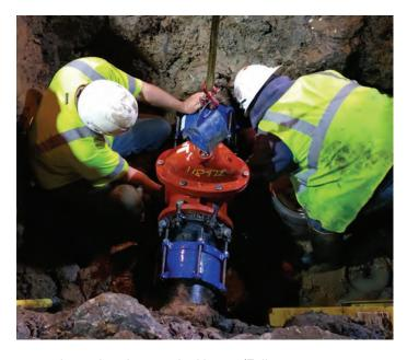
Water operators also developed a unique solution to repeated main breaks near the Houser/Fulliam intersection. By installing 300' of main line at the end of West Fulliam, there are now two feeds into the subdivision, which will increase reliability and flow. Previously, a main break could leave multiple customers without water. The timing for this upgrade was great as there are now an additional 63 lots being developed in the affected area.
