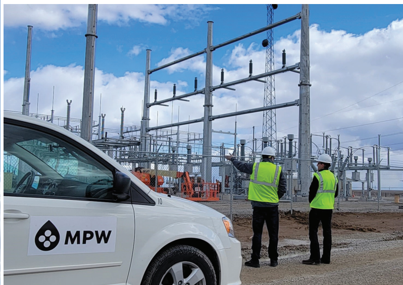
Massive steel poles, like the one shown at left carry Line 106 cross-country from MPW's West Substation to the new North Substation along Highway 38 (above).
