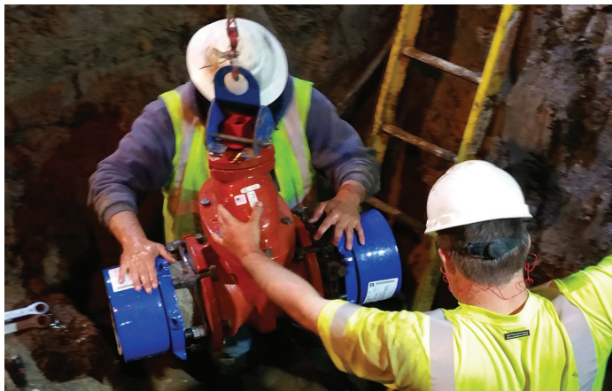
Water Distribution Operators lower a new valve into place.
