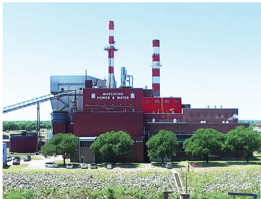
Plant 1 houses Units 7 and 8 will continue to operate as peaking units in 2023.
