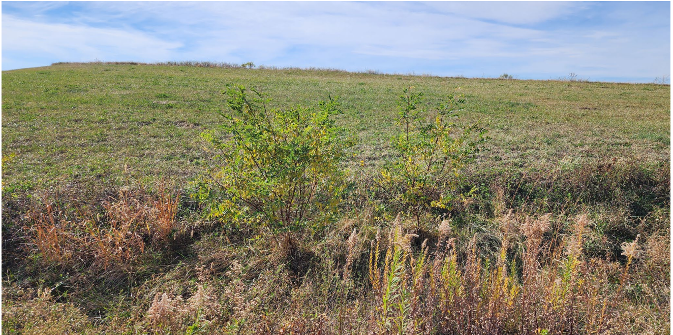
Photo 3 Example of woody vegetation growing along perimeter drainage channel and mowed final cover.
