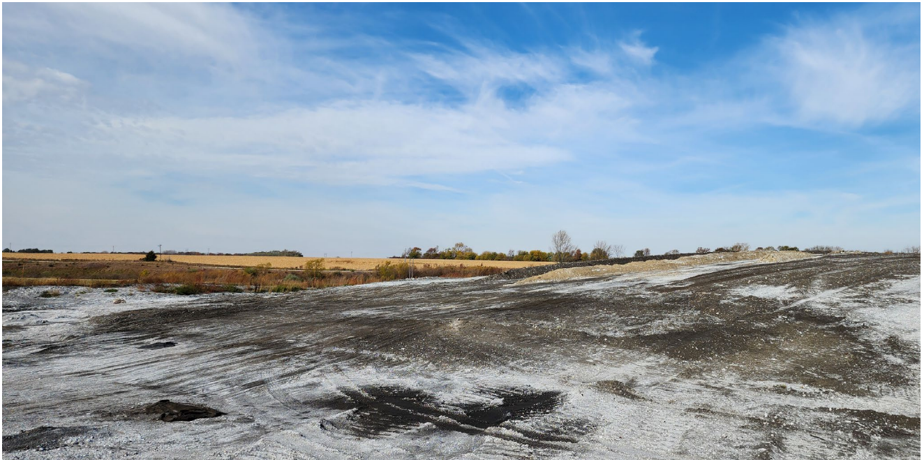
Photo 6 Active fill area showing compacted CCR and ridge of recently deposited CCR.
