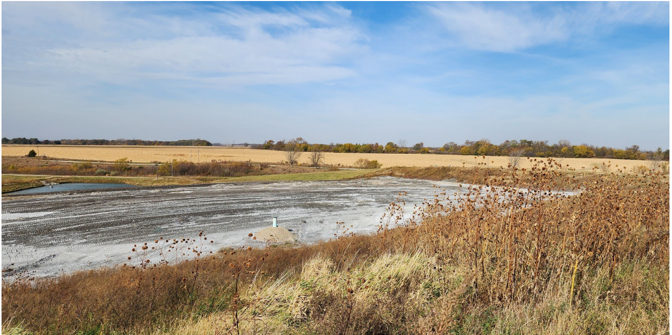
Photo 5 Active fill area looking west from access road.
