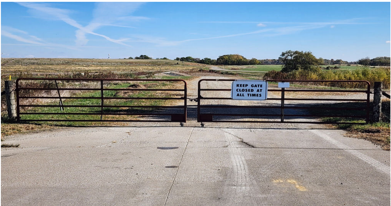
Photo 6 Typical locked entrance gate condition. Looking east.
