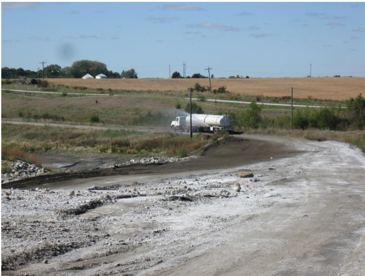
Picture 1: Water Tanker Truck wetting the haul road
