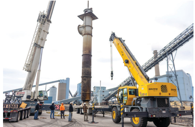
In November 2025, a Circulating Water Pump is lifted for refurbishment, part of MPW's commitment to reliable, efficient power for years to come.
