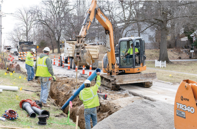
MPW Water crews replace a water main on Roscoe Street, coordinating with the City's West Hill Sewer Separation Project to minimize disruption and maximize efficiency.
